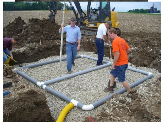
Turn surface water drains into blind inlets
